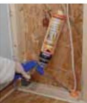
Closed cell polyurethane sealant, provides an R-value of 4-5/inch. Orange colored for easier ID by codes officials.
